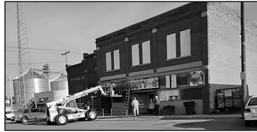
Taking down the old sign was the first big job.
